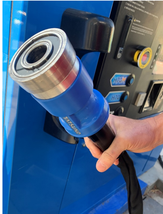
Photo 1: Hydrogen Fuel Pump Station
