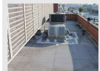
Current condition of the Fire Station 55 roof
