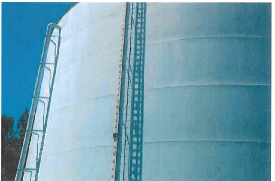
E-13 Same as Photo E-12, except further down the ladder and LLI gauge board.
