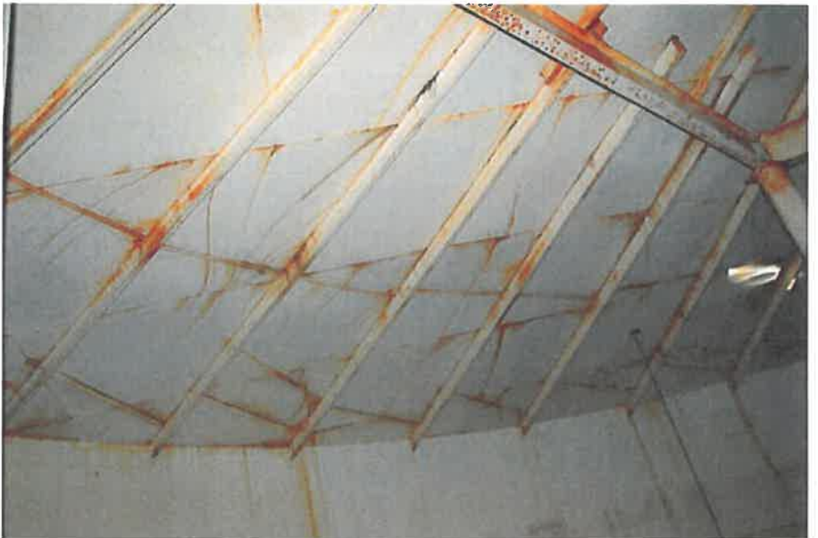
I-6 View of a portion of the outer bay, illustrating minor to moderate corrosion along the roof lap joints and lateral straps.
