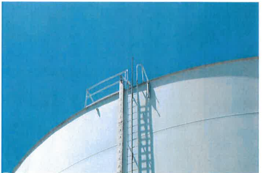
E-12 View of the upper portion of the ladder and liquid level indicator (LLI) gauge board, illustrating generally good condition of the paint system and aluminum gauge board.
