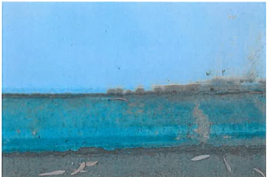
E-27 View of the bottom plate extension (BPE), illustrating moderate corrosion along the edge of the BPE.
