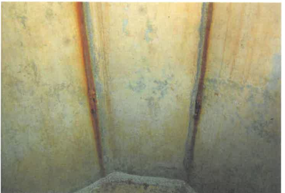
I-28 Same as Photos I-25 through I-27, except in a different location.
