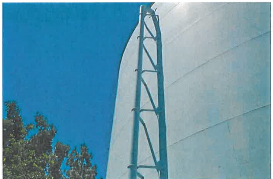
E-16 Same as Photo E-15, except further down the pipe.
