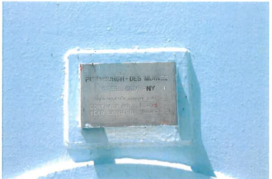
E-26 View of the identification (ID) plate, illustrating good condition of the plate.
