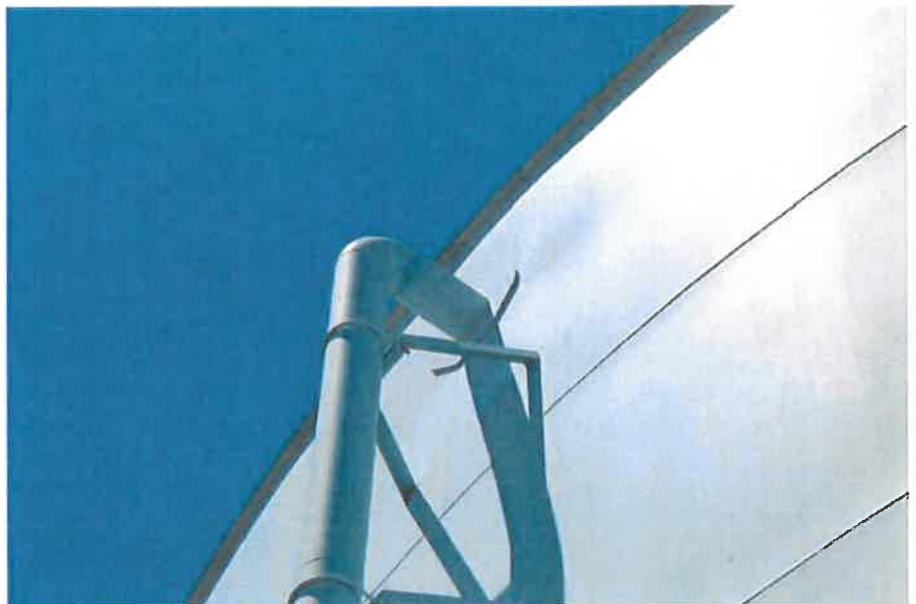
E-15 View of the upper portion of the overflow pipe, illustrating good condition of the paint system.
