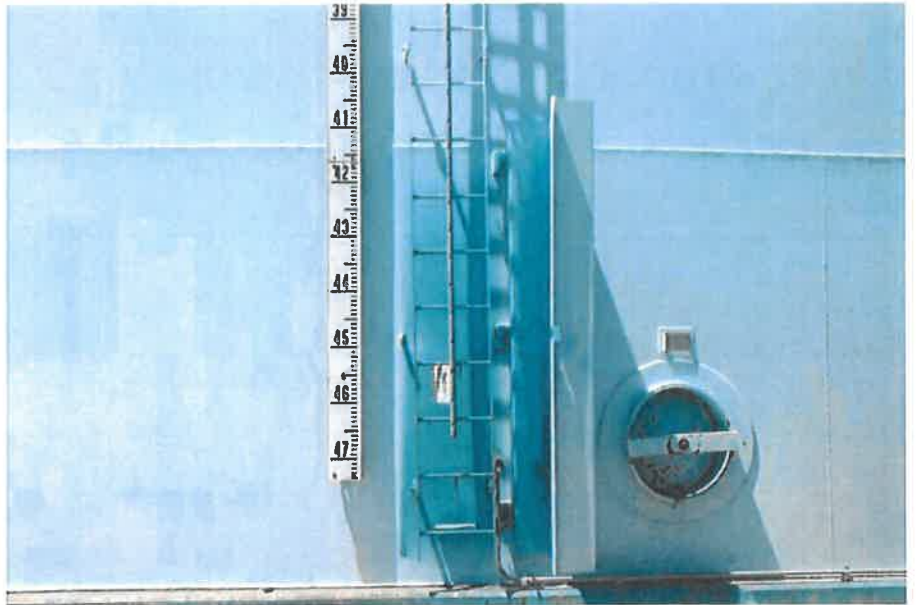
E-14 Same as Photos E-12 and E-13, except at the bottom of the ladder.
