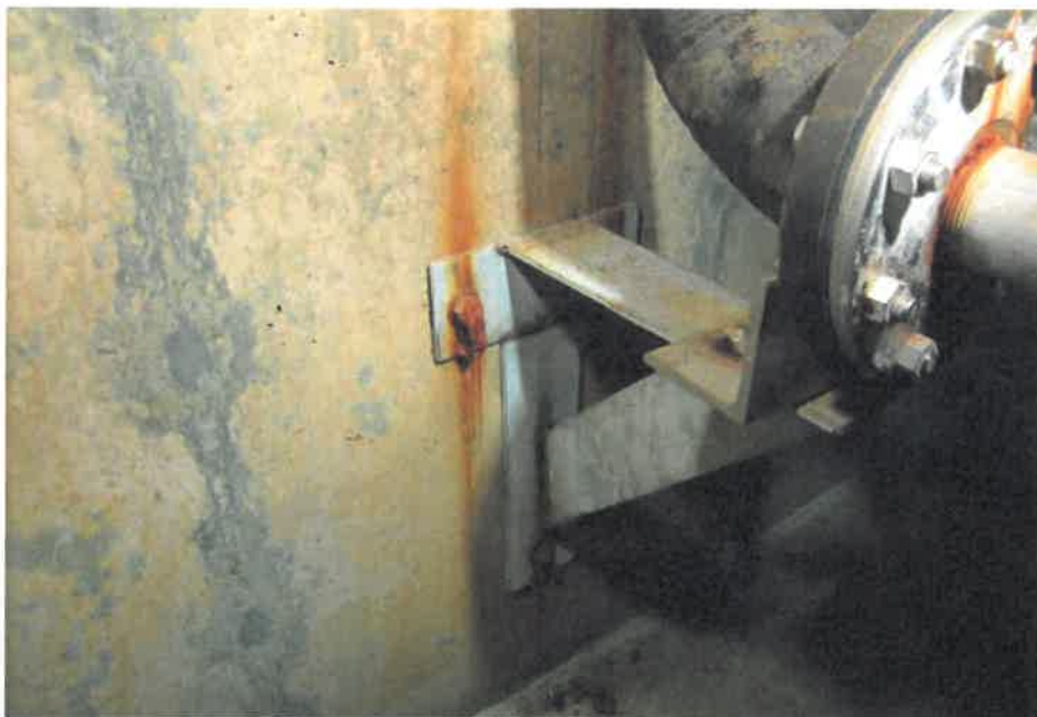
I-33 Same as Photos I-30 through I-32, except in a different location.
