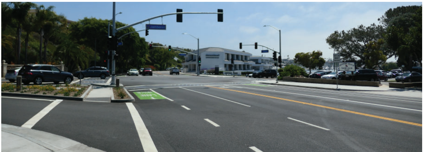
Multimodal Improvements on Bayside Drive, Newport Beach
