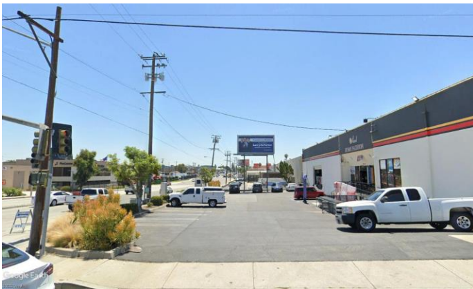
Existing West Face
