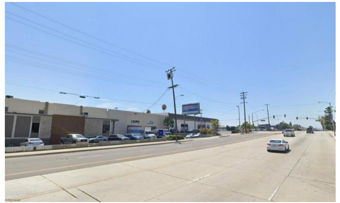
Existing East Face
