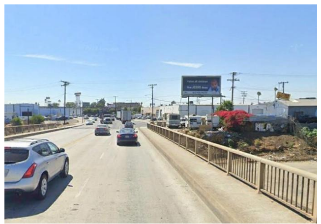
Existing East Face
