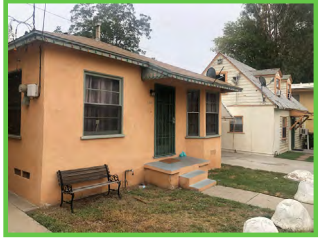
South elevation of 132 N Poplar Ave
