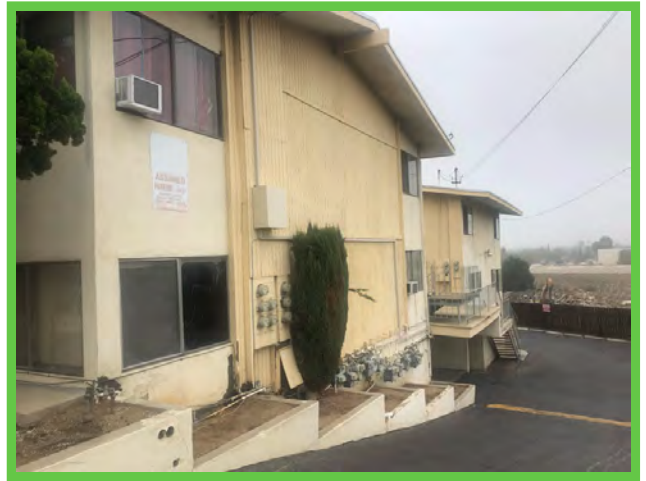
South elevation of 116 Poplar Ave
