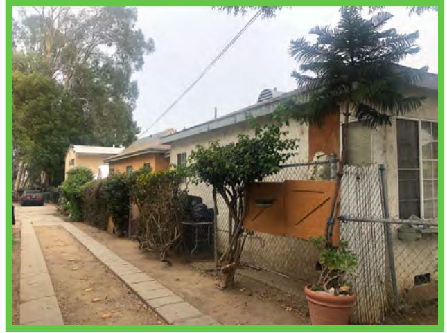
South elevation of 136 N Poplar Ave 16
