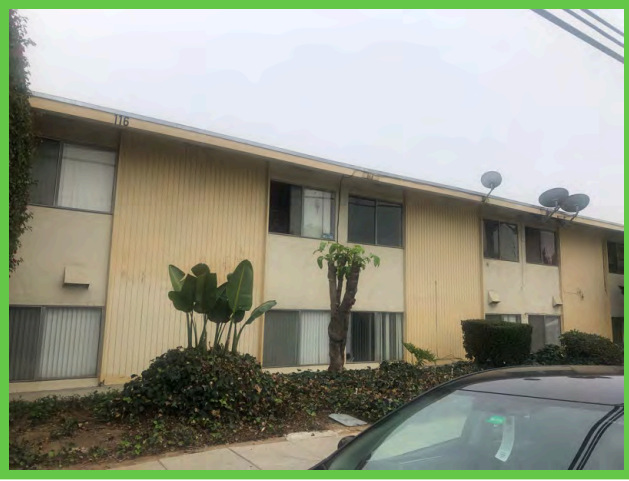
Front view of 116 Poplar Avenue facing West
