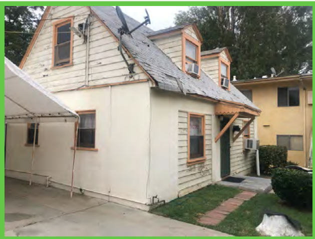
South elevation of 134 N Poplar Ave
