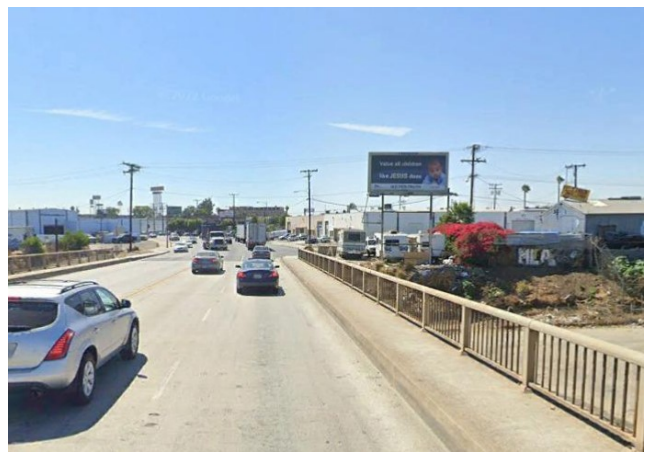
Existing East Face
