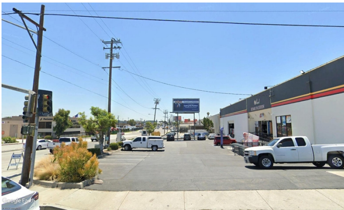
Existing West Face
