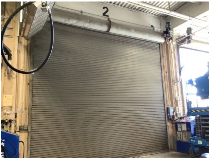
16' x 14', Cookson, Maintenance shop 2/13/2023 10:19 AM
