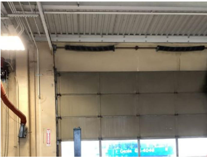
14' 2" x 12', Sectional door, Mainten... 2/13/2023 3:31 PM
