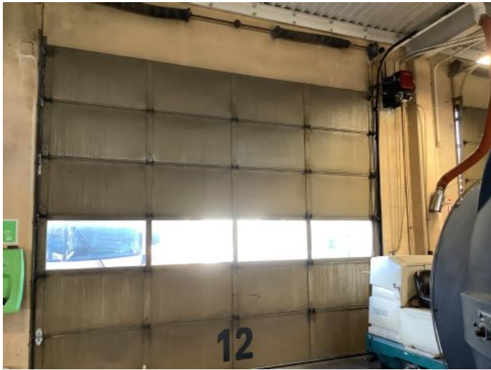
14' 2" x 12', Sectional door, Mainten... 2/13/2023 3:26 PM VIEW
