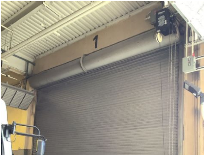
16' x 14', Cookson, Maintenance shop 2/13/2023 10:14 AM
