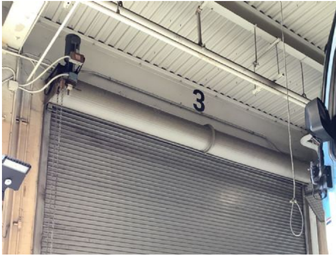
16' x 14', Cookson, Maintenance shop
