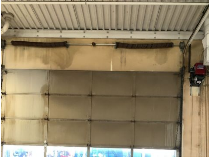
14' 2" x 12', Sectional door, Mainten... 2/13/2023 3:16 PM
