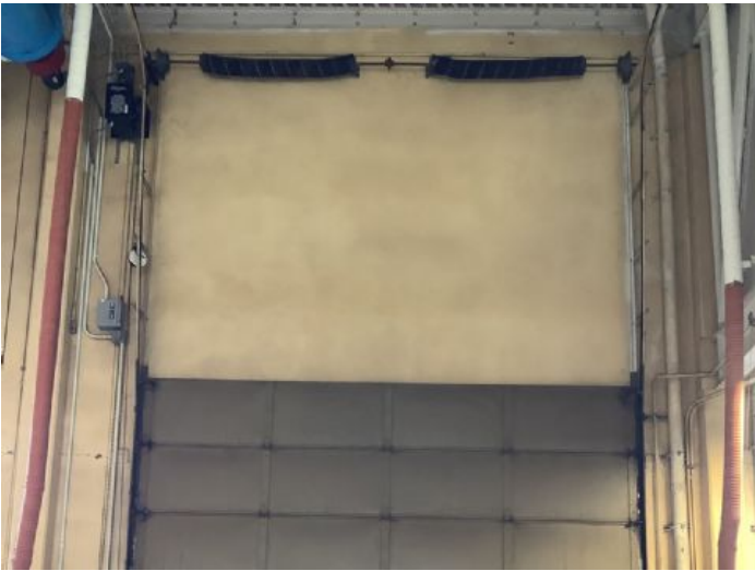
14' 2" x 14', Sectional door, Mainten... 2/13/2023 3:12 PM
