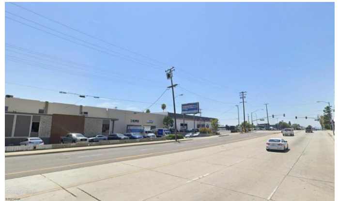
Existing East Face
