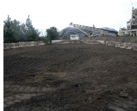
Lead-impacted soil from former trap shooting operation was excavated, treated and disposed.
