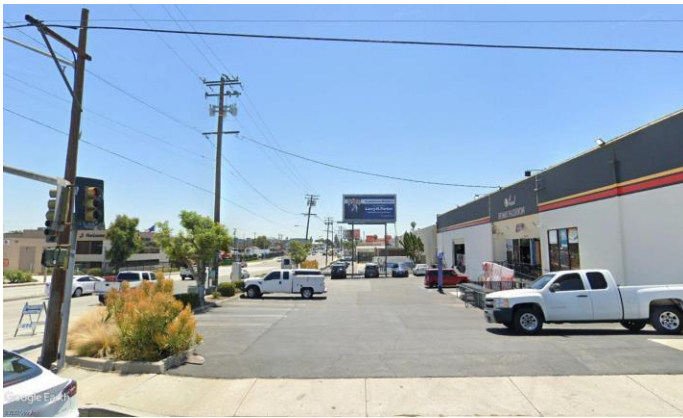
Existing West Face
