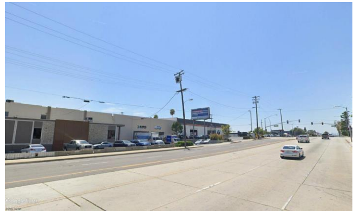
Existing East Face
