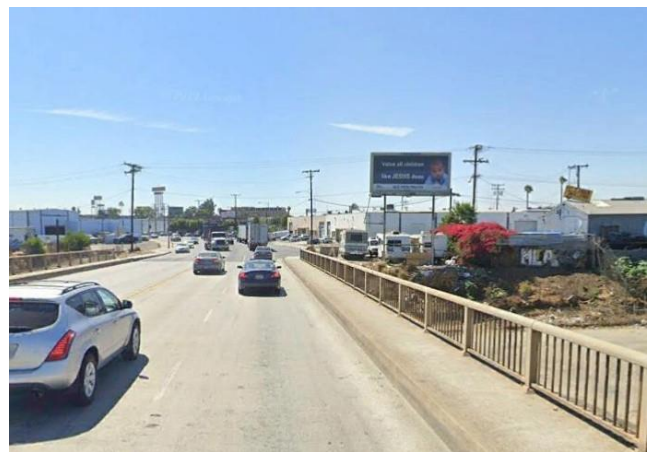
Existing East Face
