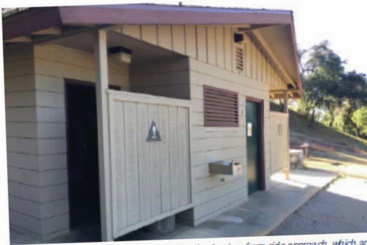
Drinking fountain does not have cane detection barriers from side approach, which are required if the fountain is not located within an alcove.
