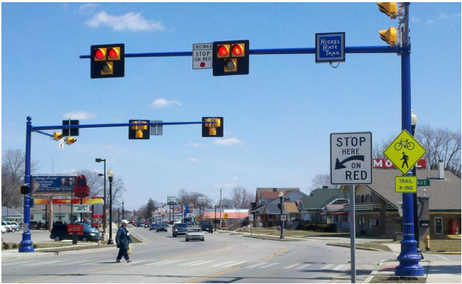
Signals and Warning Devices
