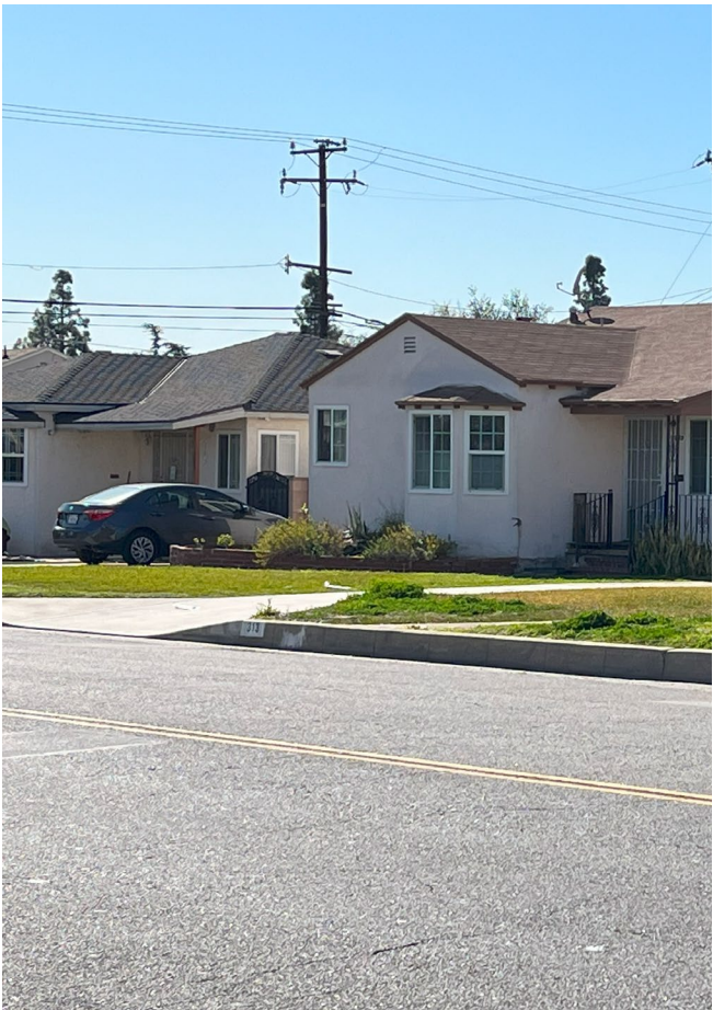
Inconsistent sidewalk gaps on Wilcox Avenue
