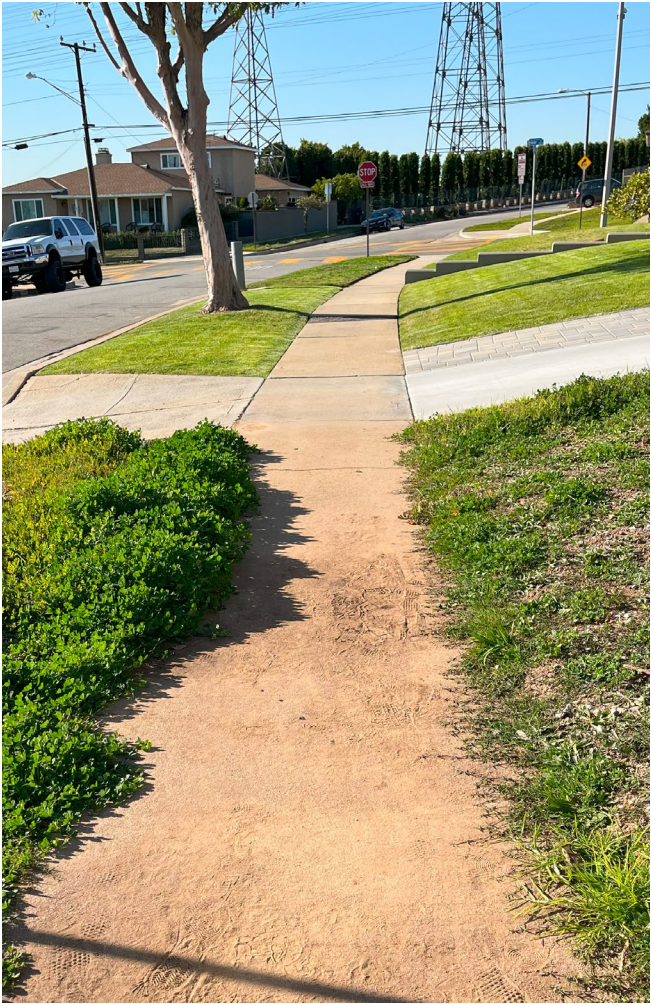
Sidewalk missing or covered with dirt on Lincoln Avenue
