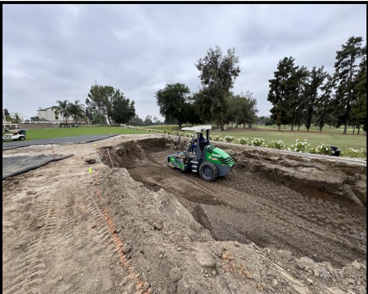
Sheep's foot roller compacting soil
