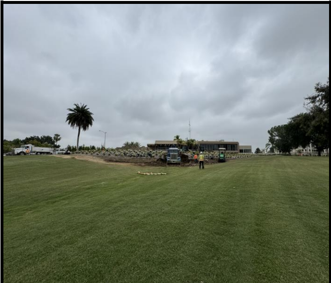
Loading up saturated soil for transportation to golf course
