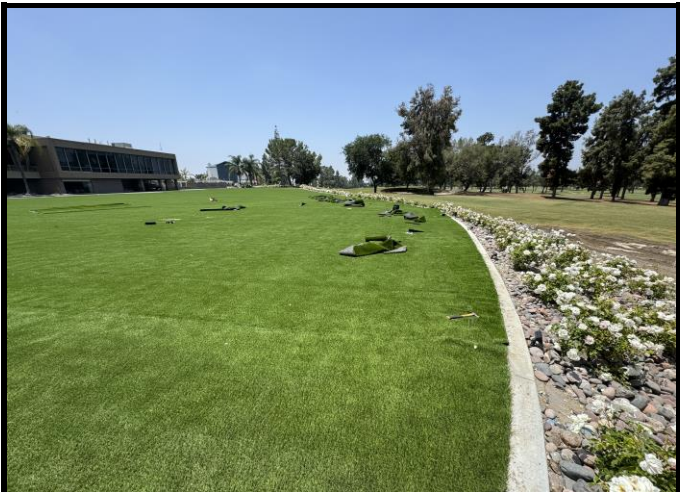
Laguna cutting off strips of turf to help bridge gap between turf and curb
