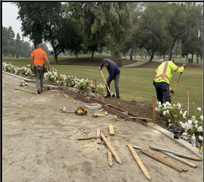
Saldana forming up in preparation for the concrete pour of curb
