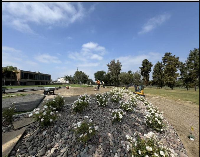
Saldana performing small touch ups of hillside
