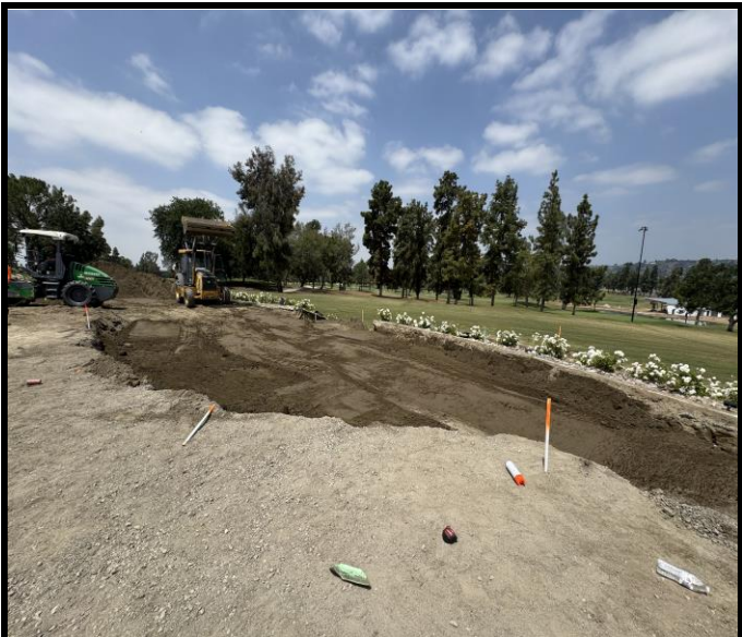
Raising East side of event lawn in 8 inch lifts
