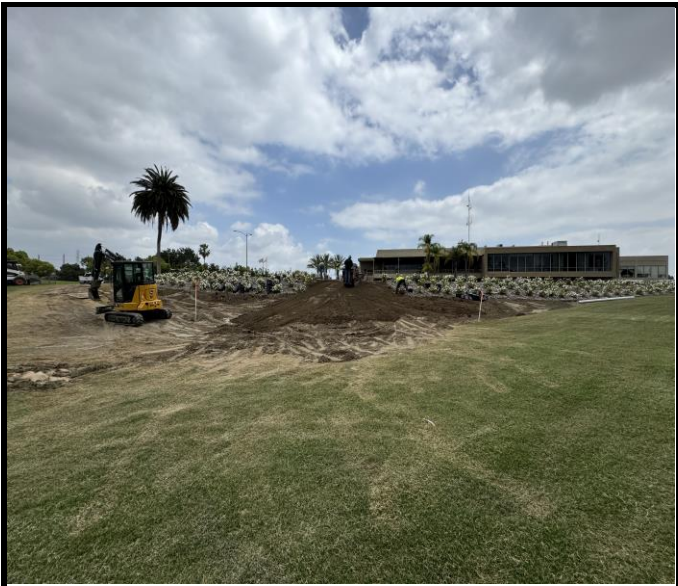
Hillside grading taking place.
