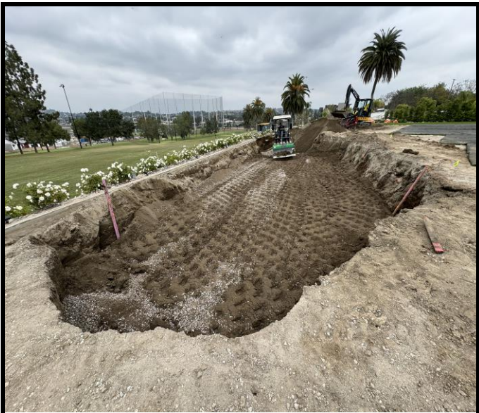
Compaction and 8 inch lifts continue
