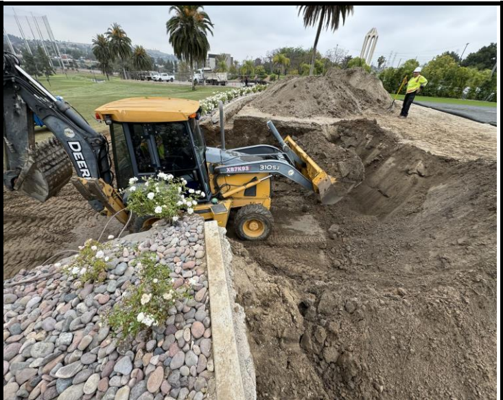
Excavation until contractor reaches native
