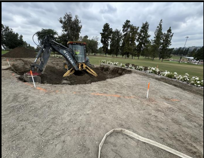
Excavation on east side of event lawn begins. Saldana aims to reach native ground
