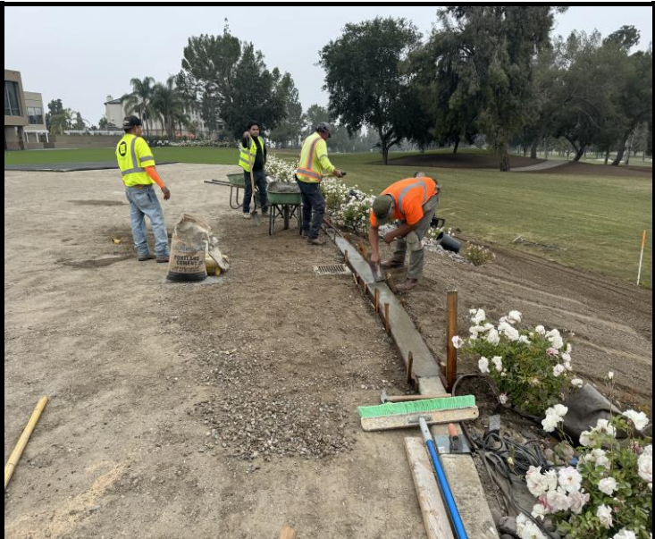
Concrete curb poured.
