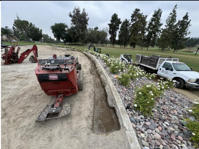
Saldana trenching for drainage line along curb
