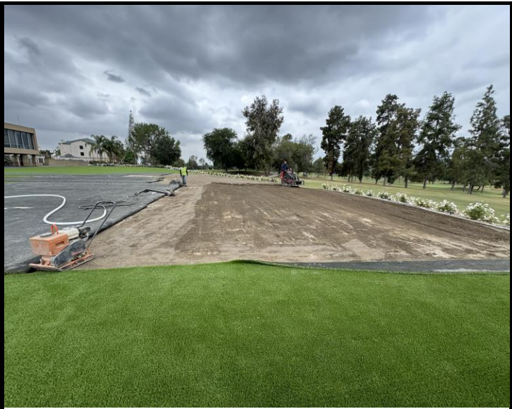
Event lawn grading taking place in preparation for Laguna Turf return next week
