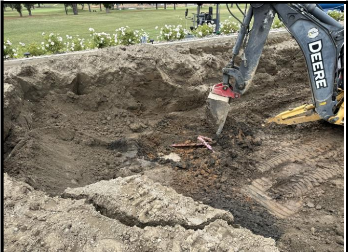
Abandoned Water line hit at 2:30 pm and afterwards line was cut and capped
