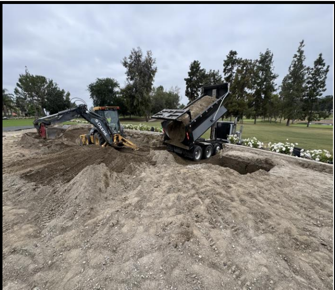
Saldana receiving imported soil to bring west side of event lawn up to its proper grade
