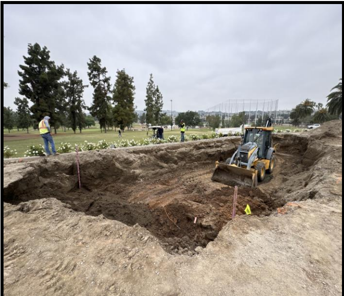
Saldana reaches native and is ready to start bringing up soil to grade in 8 inch lifts
