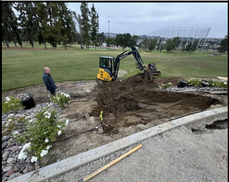
Excavation of slope continues
