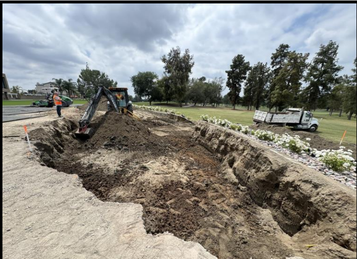
East side excavation progress
