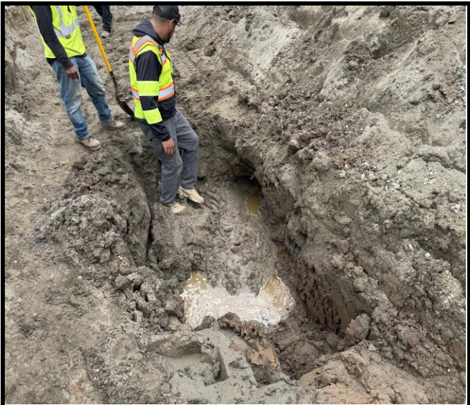
Water pocket found while excavating
