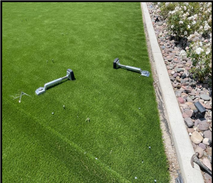
Laguna rolls back Turf but is short of the curb by about 2-3 inches due to shrinkage
