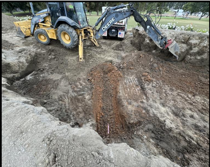
Abandoned irrigation line discovered just above native ground. Pipe was cut and capped.
