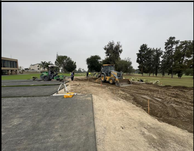
Saldana fiinishing up final grading of soil before base is place's at
