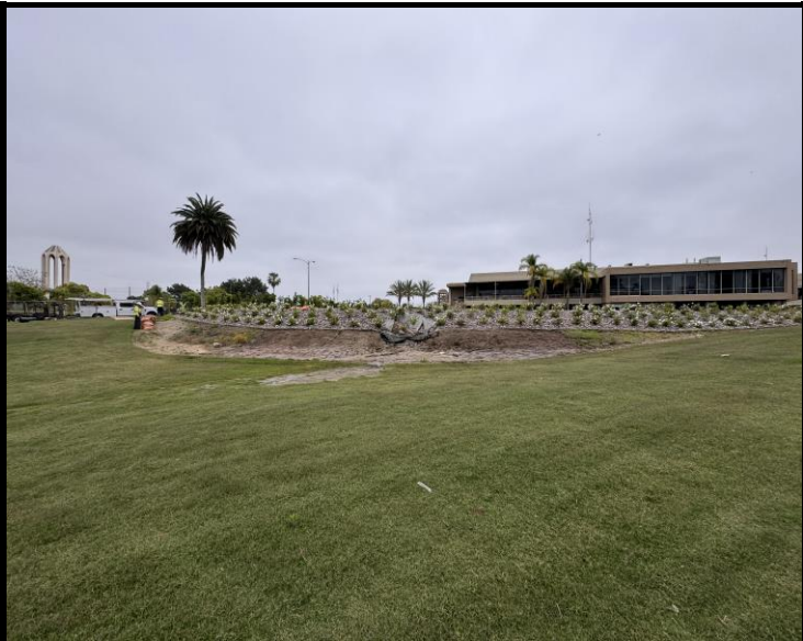
Collapsed slope of event lawn
