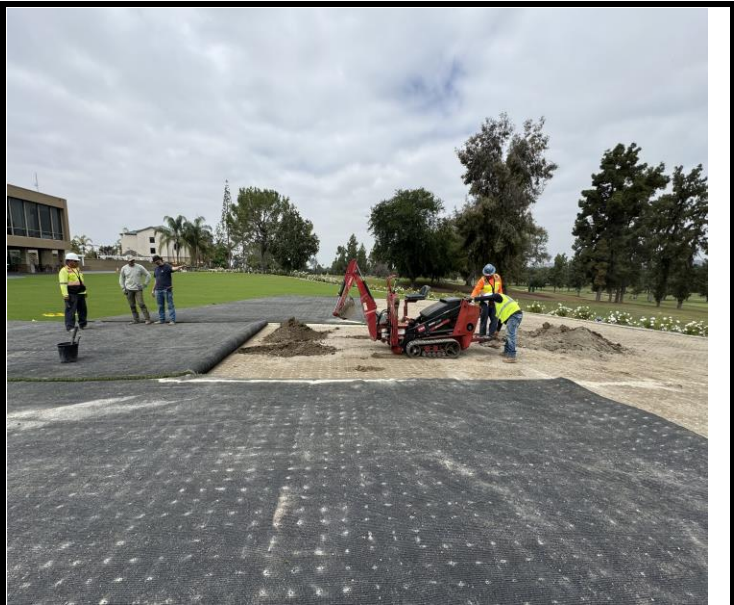
Saldana chasing saturated solid to determine the extent of compromised soil
