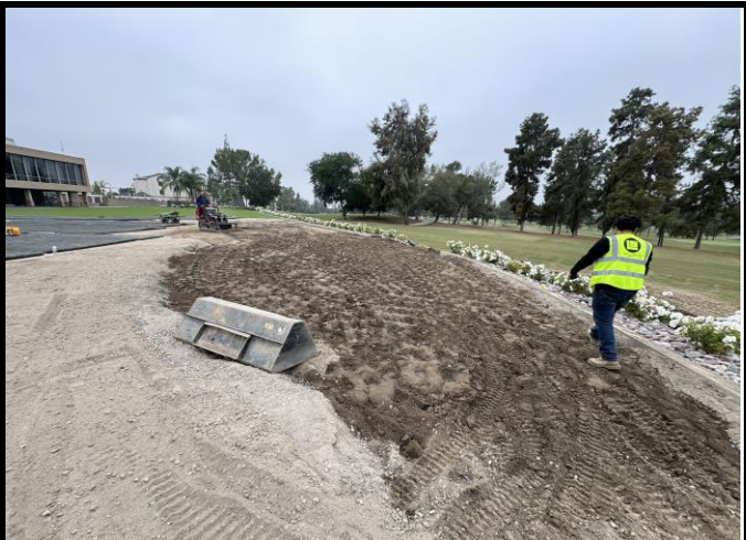
Event lawn soil fully compacted and ready for 5 inches of base
