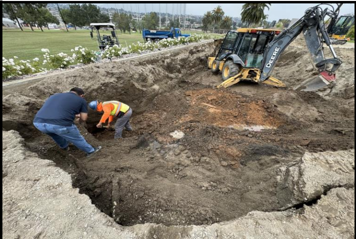
Excavation of saturated soil continues until native is reached
