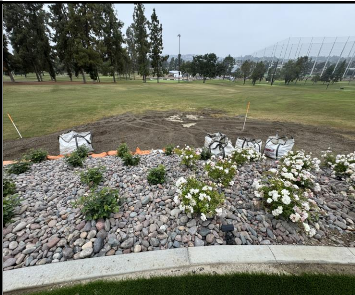
Saldana not on site today. Hillside temporarily restored until 12 inch drainage pipe can be installed
