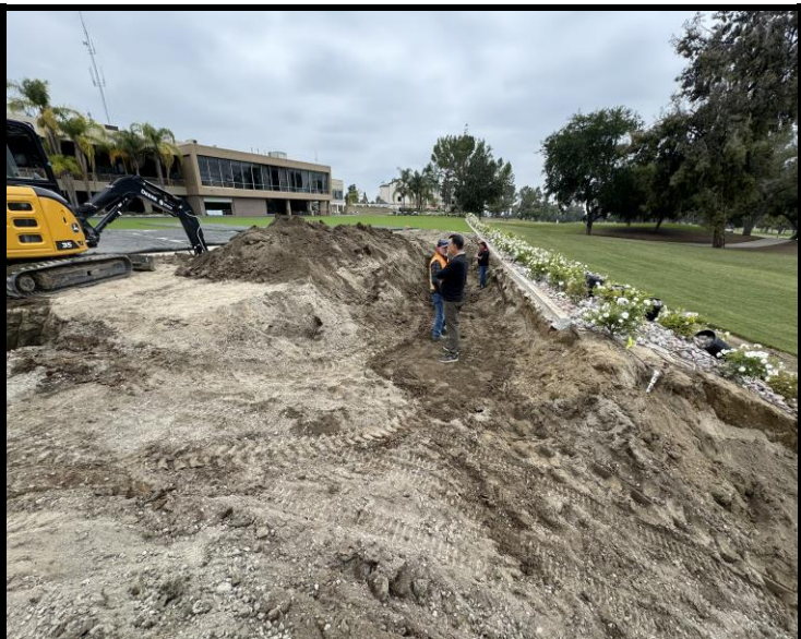
Excavation of 2 feet to find suitable compacted ground
