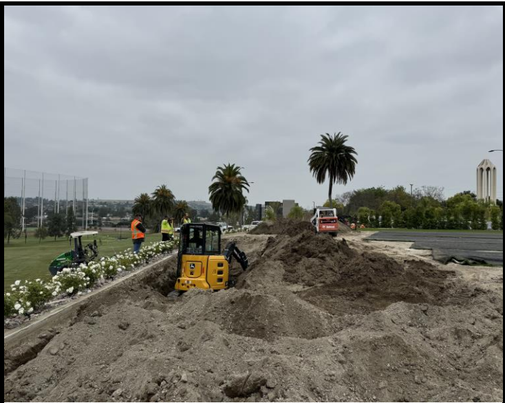
Excavation of saturated soil continues
