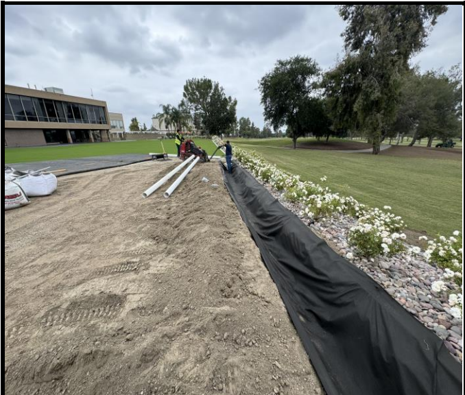
Saldana trenching out drainage line
