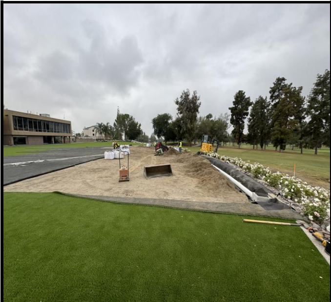
Saldana continues installing drainage line
