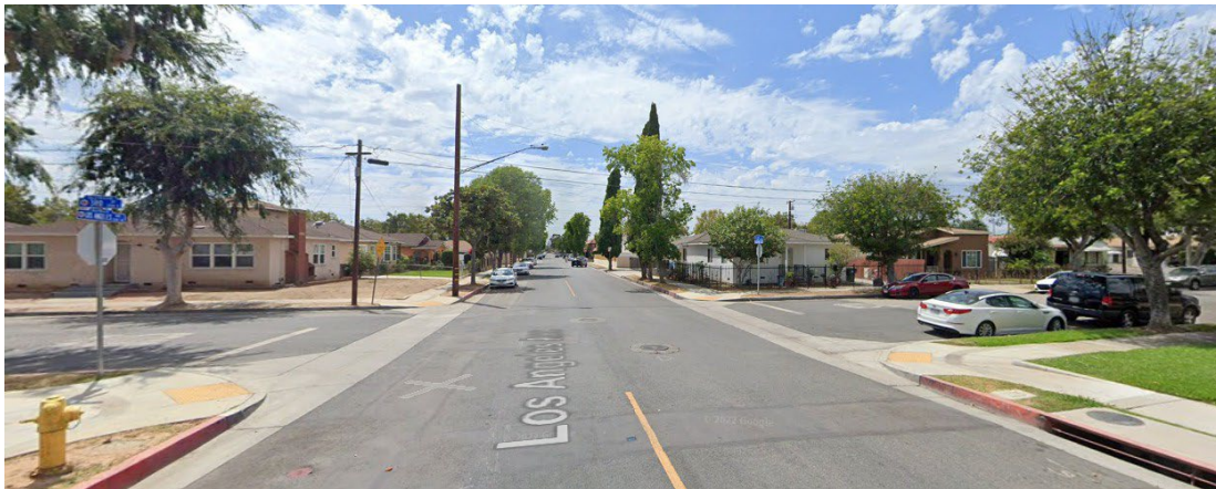
Figure 5 - Street View of 3rd Street at Los Angeles Avenue, Looking East
