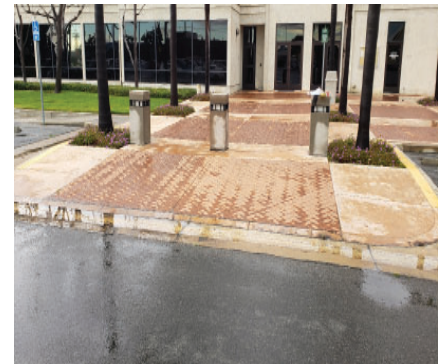
JWA ADA Improvements
