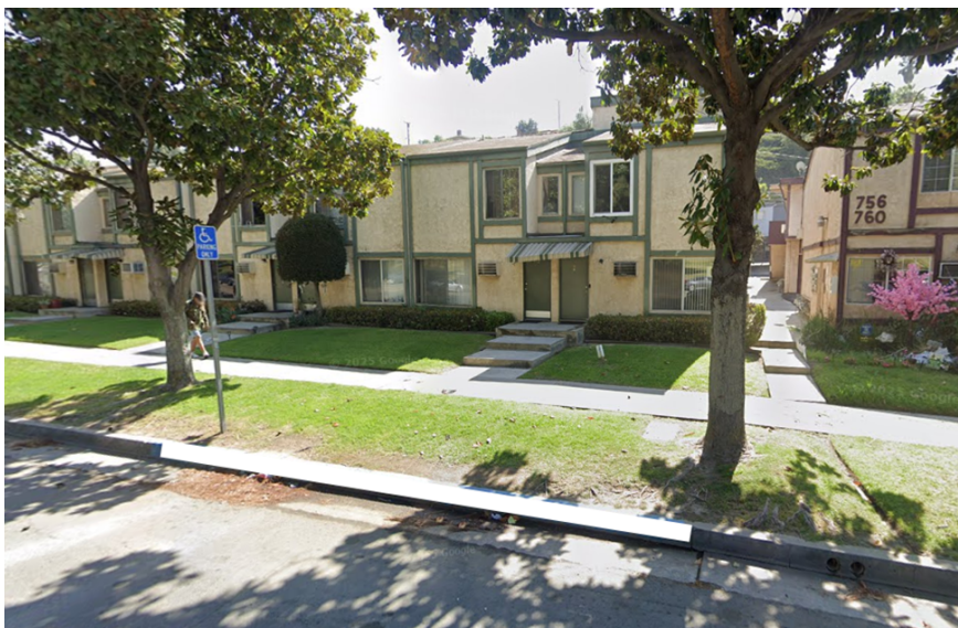
Figure 3 - Recommended Blue Curb Removal at 764 N. Garfield Avenue
