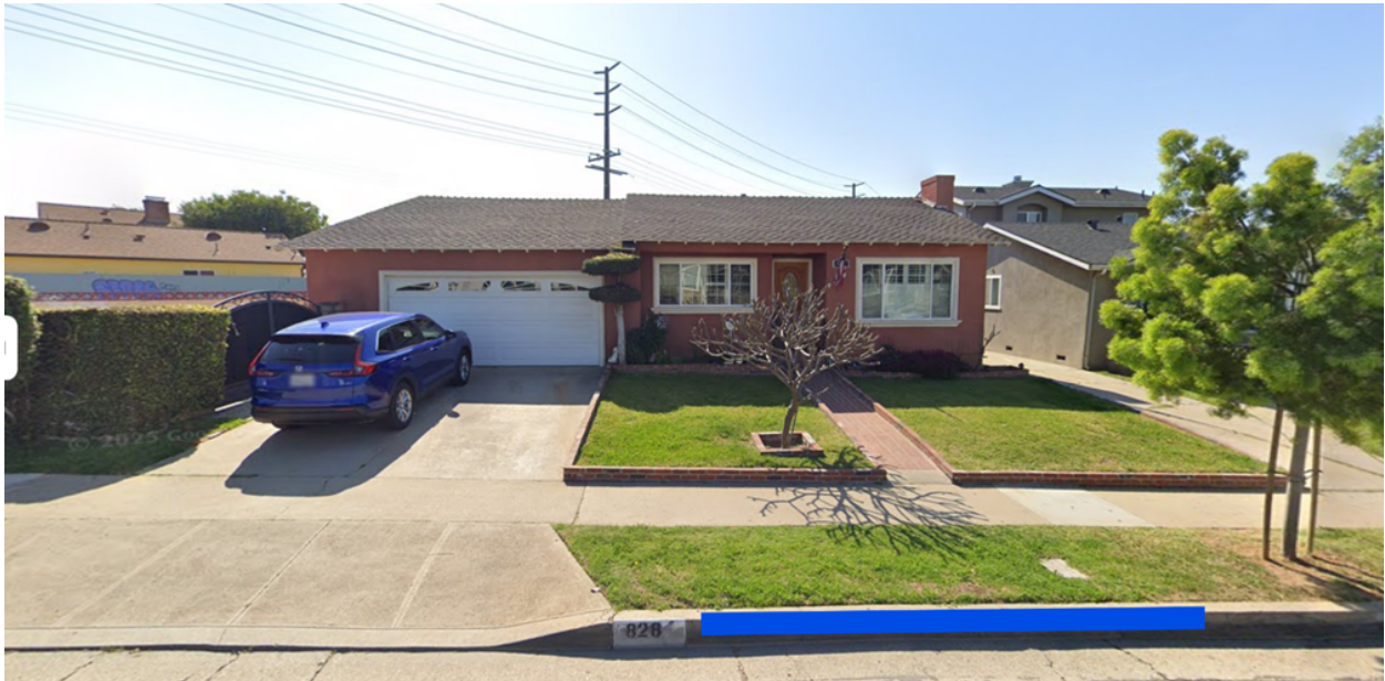
Figure 3 - Recommended Amount of 15 Feet of Blue Curb Fronting 828 North Hay Street
