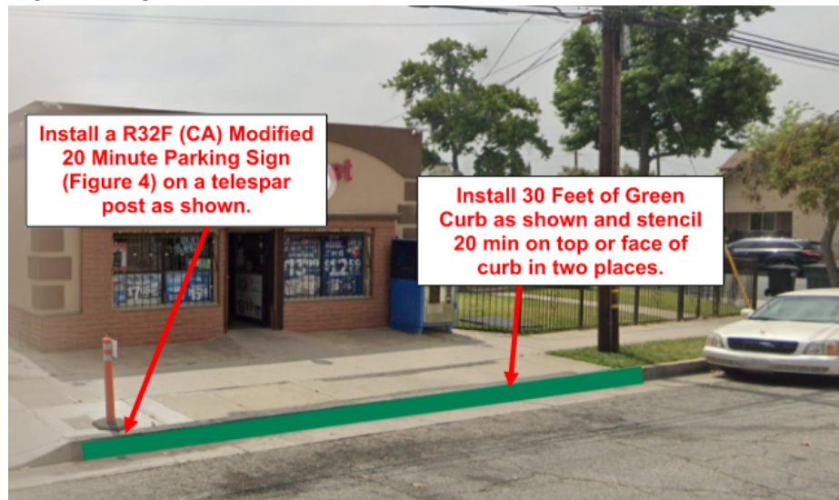
Figure 3 – Installation of 30 Feet of Green Curb Fronting 140 South 5 th Street.
