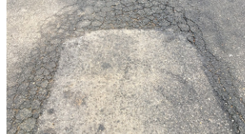
PCI 0-40 (Very Poor/Failed)
