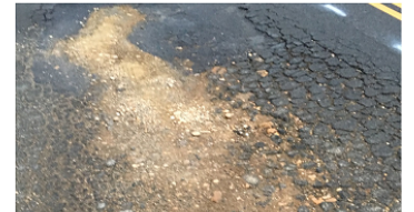
PCI 0-40 (Very Poor/Failed)
