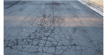
PCI 0-40 (Very Poor/Failed)
