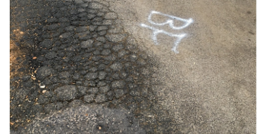
PCI 0-40 (Very Poor/Failed)
