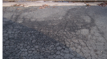
PCI 0-40 (Very Poor/Failed)
