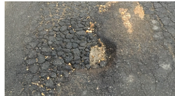
PCI 0-40 (Very Poor/Failed)
