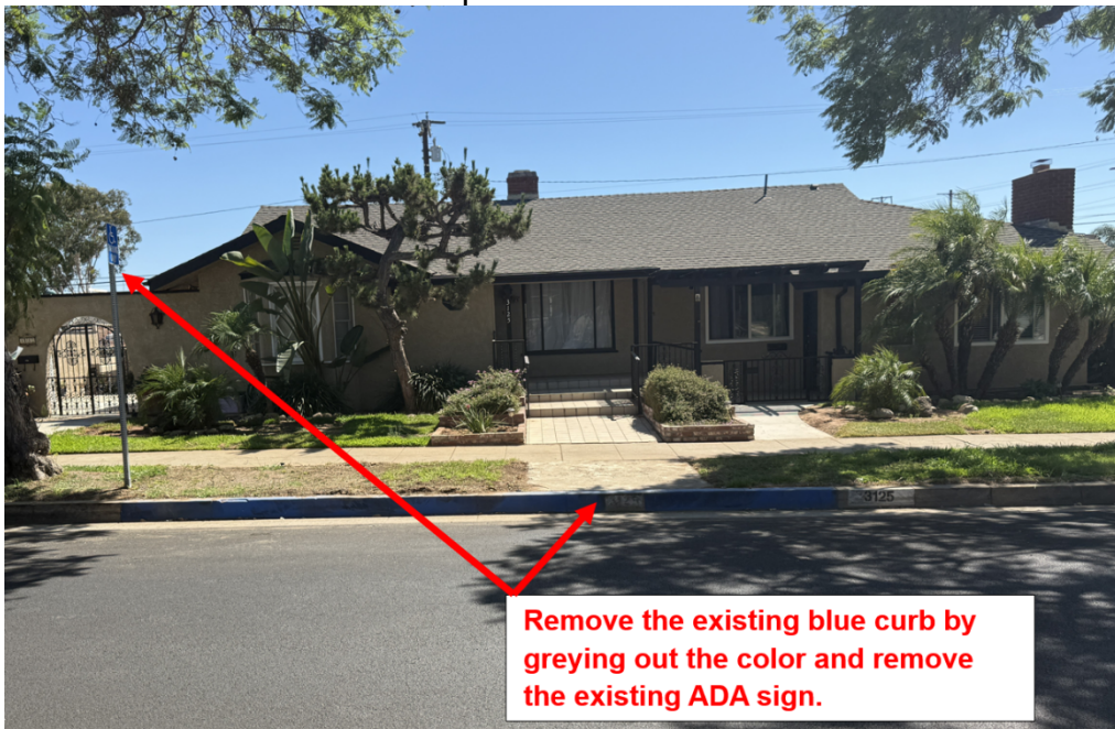
Figure 3 – Recommended Blue Curb Removal at 3125 Via San Delarrio
