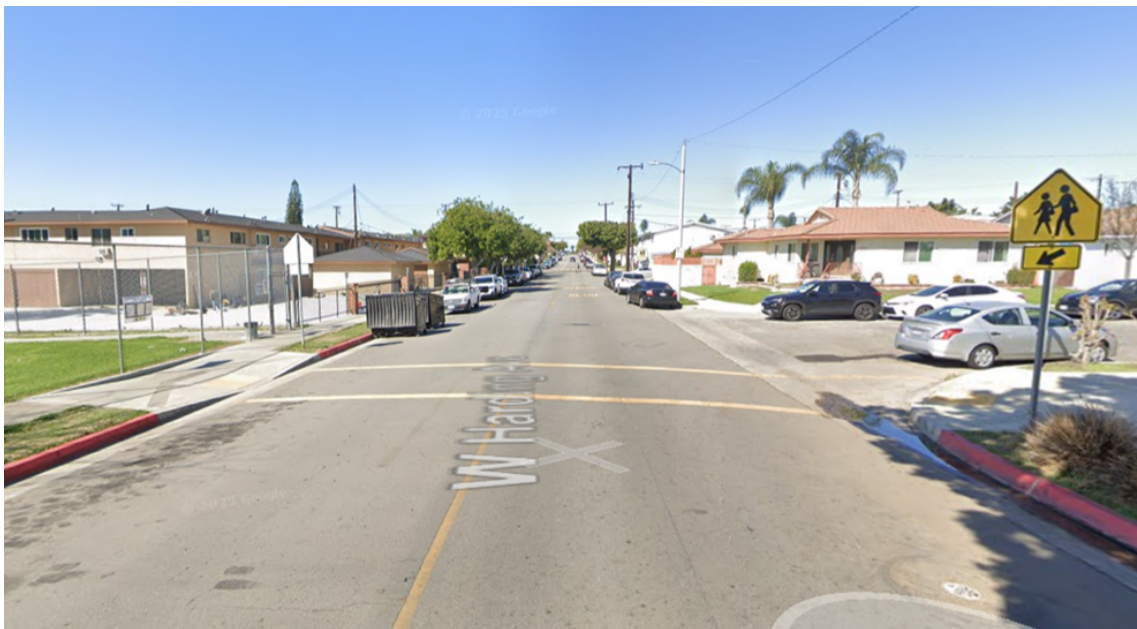
Figure 2 - Street View of West Harding Ave at North Park Ave Looking West on West Harding Ave
