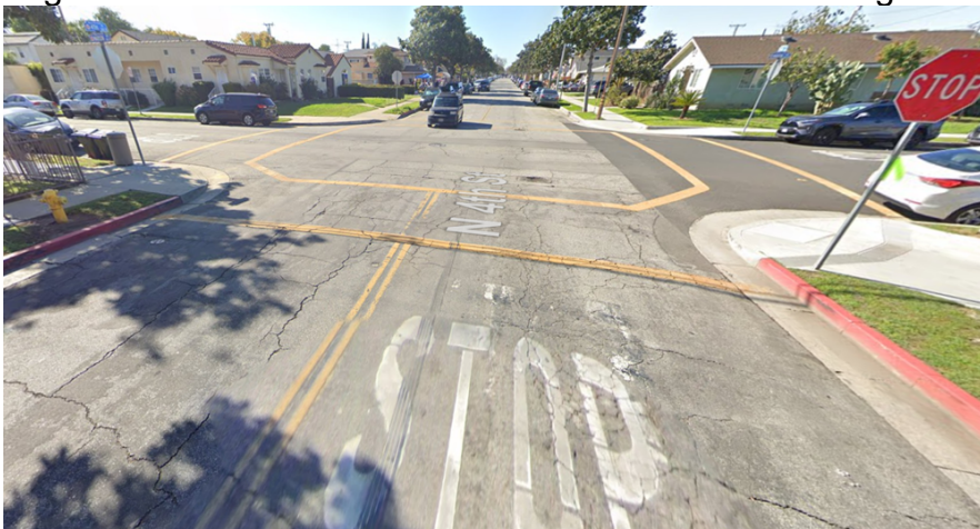
Figure 4 – Southern View of N 4th Street Looking at W Madison Avenue
