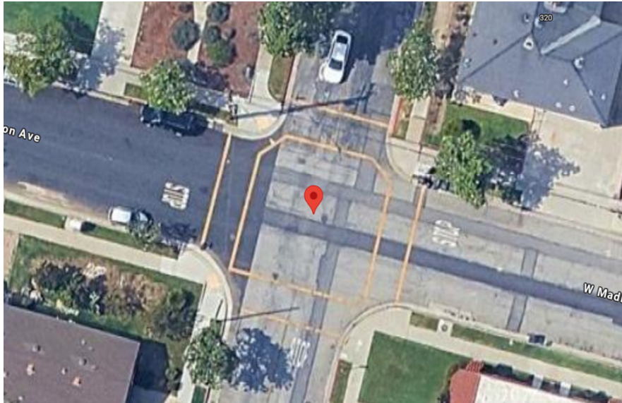
Figure 1 – Aerial View of W Madison Avenue and N 4th Street
