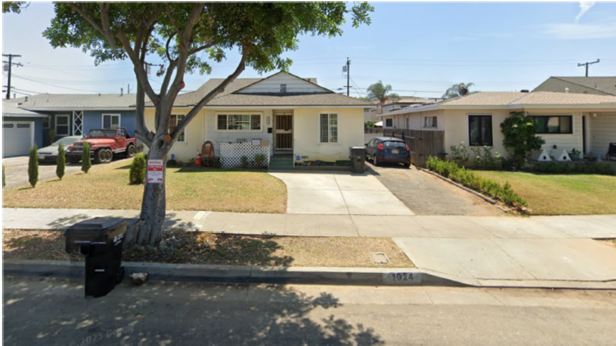
Figure 2 - Street View of 1024 S 4 th Street Looking East.
