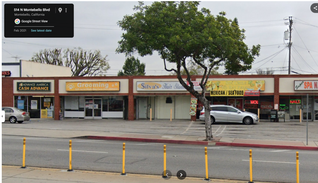
Figure 1: Curb in front of 512 N. Montebello Blvd. has been red since February 2021
