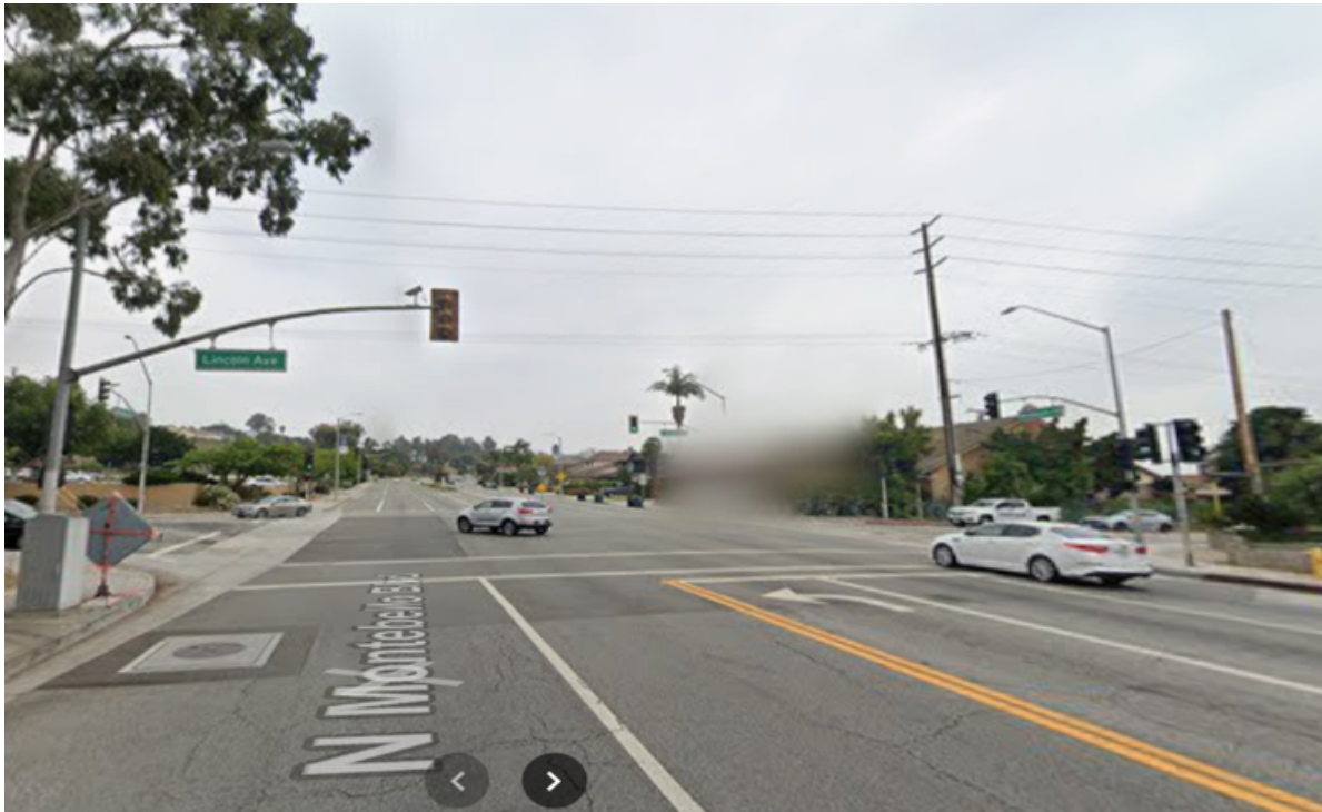
Figure 7 - Street View of N Montebello Boulevard at Lincoln Avenue
