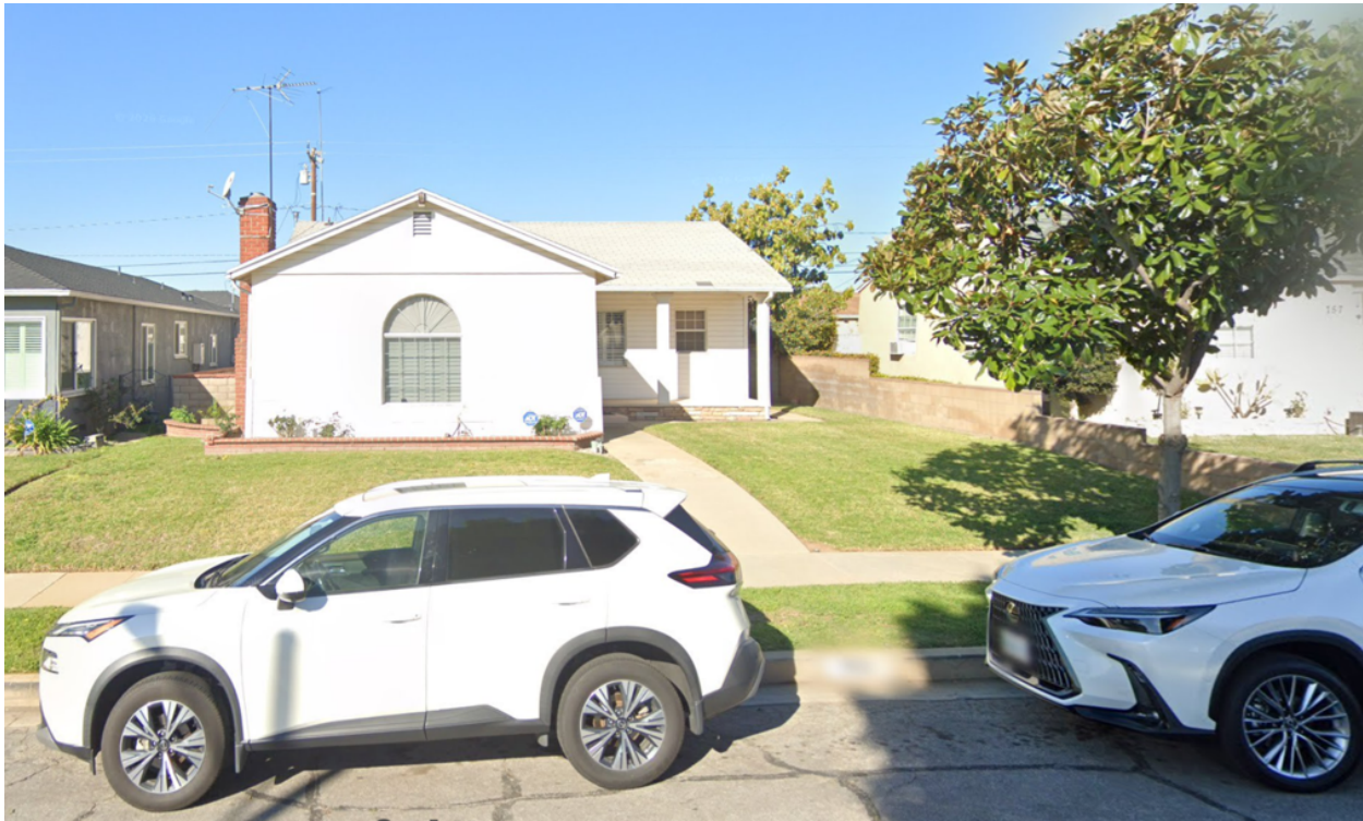
Figure 2 — Street View of 753 Bradshaw St Looking East
