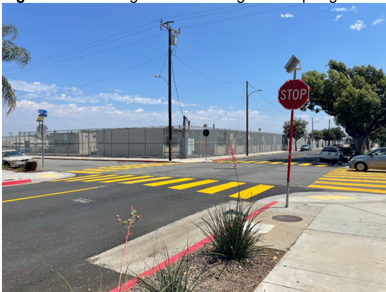
Figure 4 – N Vail Ave & W Cleveland Ave – South Bound
