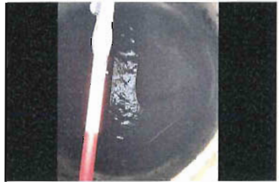
Manhole During Install
