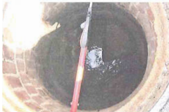
Manhole During Install
