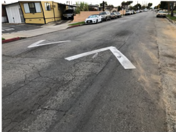
BEACH STREET: LOOKING EASTERLY (SPEED HUMP IN FOREGROUND)
