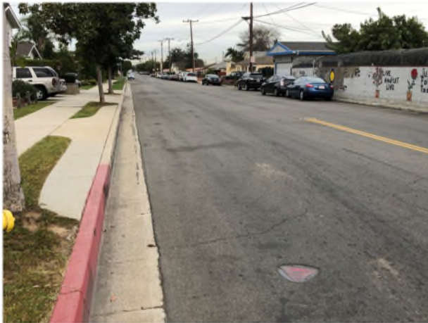
BEACH STREET: LOOKING EASTERLY (WATER VALVE IN FOREGROUND)
